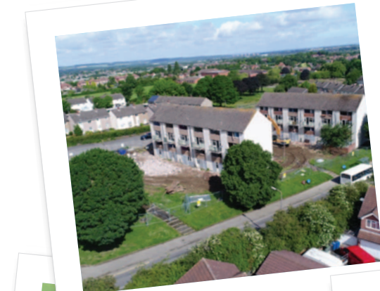
Tinkers Green demolition commences
